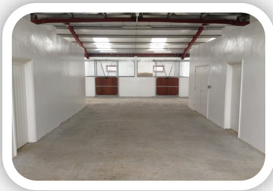
STABLES & STABLE BARN WALLS
